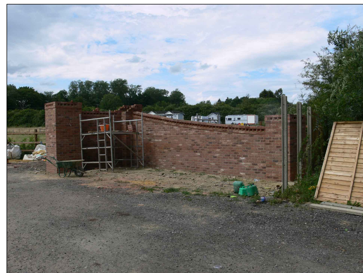
NOTE 3 - ENTRANCE WING WALLS
